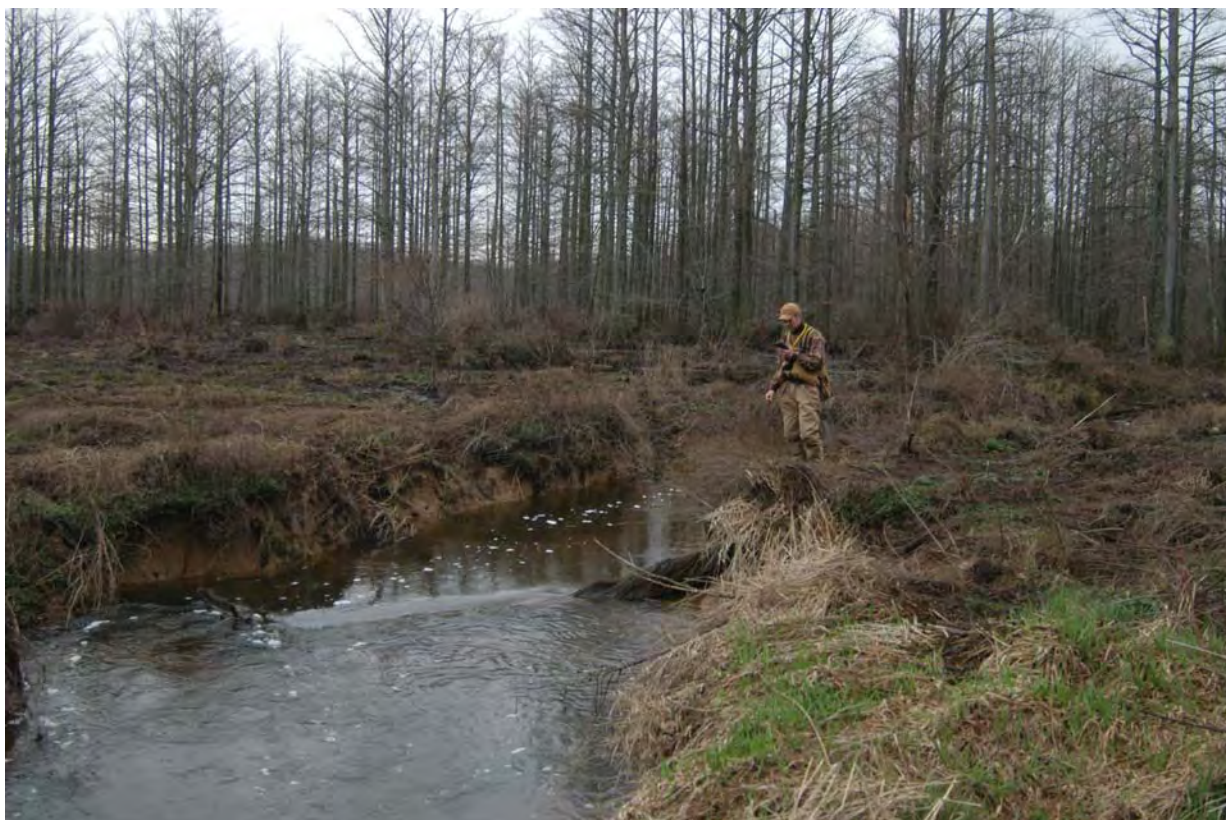
Figure 17 Looking upstream at bank erosion on Ditch 1.
