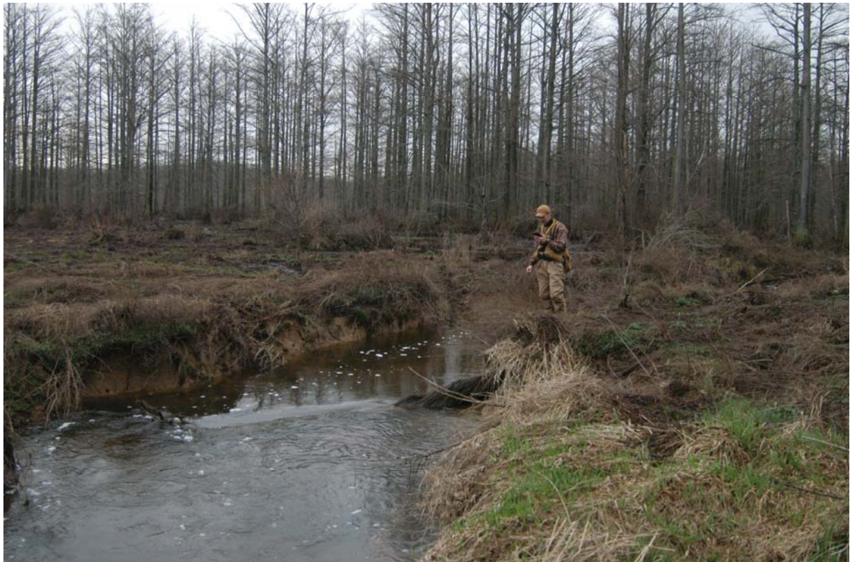
Figure 17 Looking upstream at bank erosion on Ditch 1.
