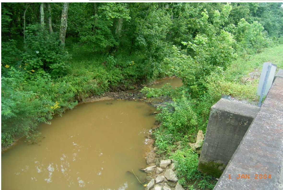
Figure 9 (Below) Little Joe Creek looking downstream along the upstream (east) side of the north KY-307 crossing.
