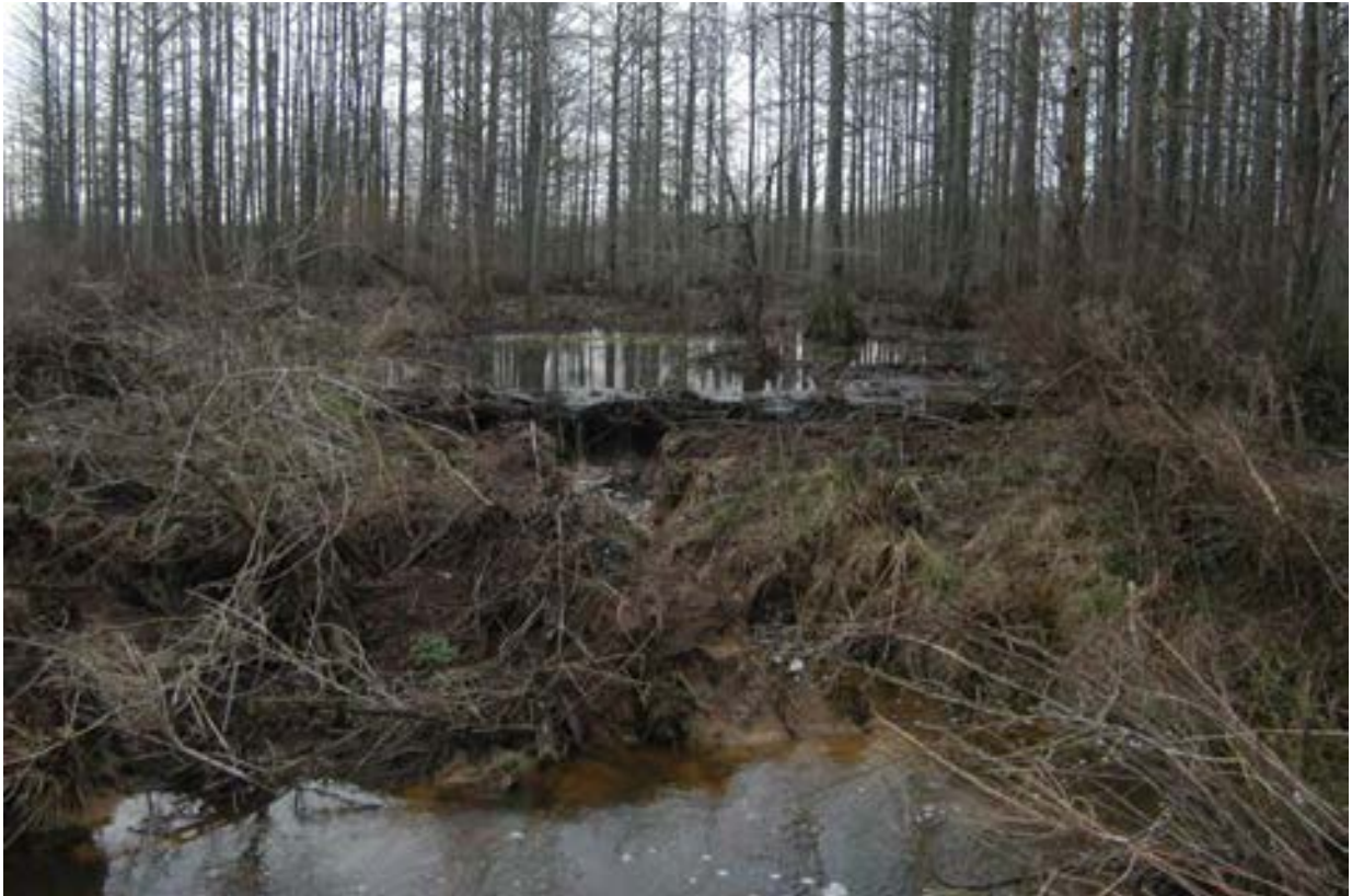
Figure 19 Turned 90° to the left from preceding photo of Ditch 1. Headcut/bank erosion from main beaver dam.
