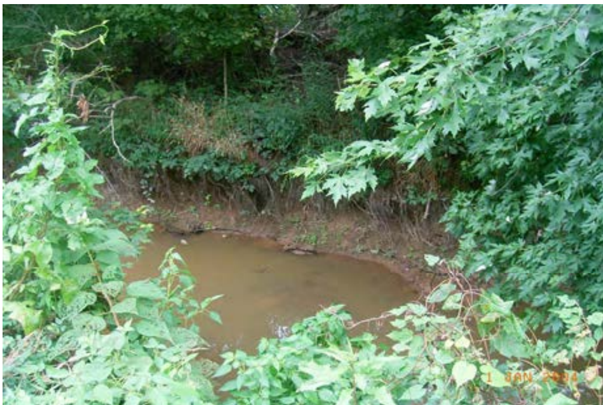
Figure 13 (Below) Little Joe Creek: Undercut bank upstream of confluence with Ditch 1.
